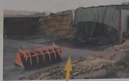
3 driving silo, 약 2700m3 저장용량
